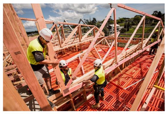
WorkDek makes standing of trusses easy and safe compared to working on ladders, and much faster than using cranes to lift and position each truss.
